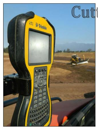
Using the Trimble GPS system to construct a new pond at Lion Mountain Ranch in Ojai is allowing C. A. Rasmussen to save money on the project by not using surveyors. (Right) Foreman Brandon Medema uses the Trimble rover to check grade as Tim Markley cuts grade without the need of survey staking.
