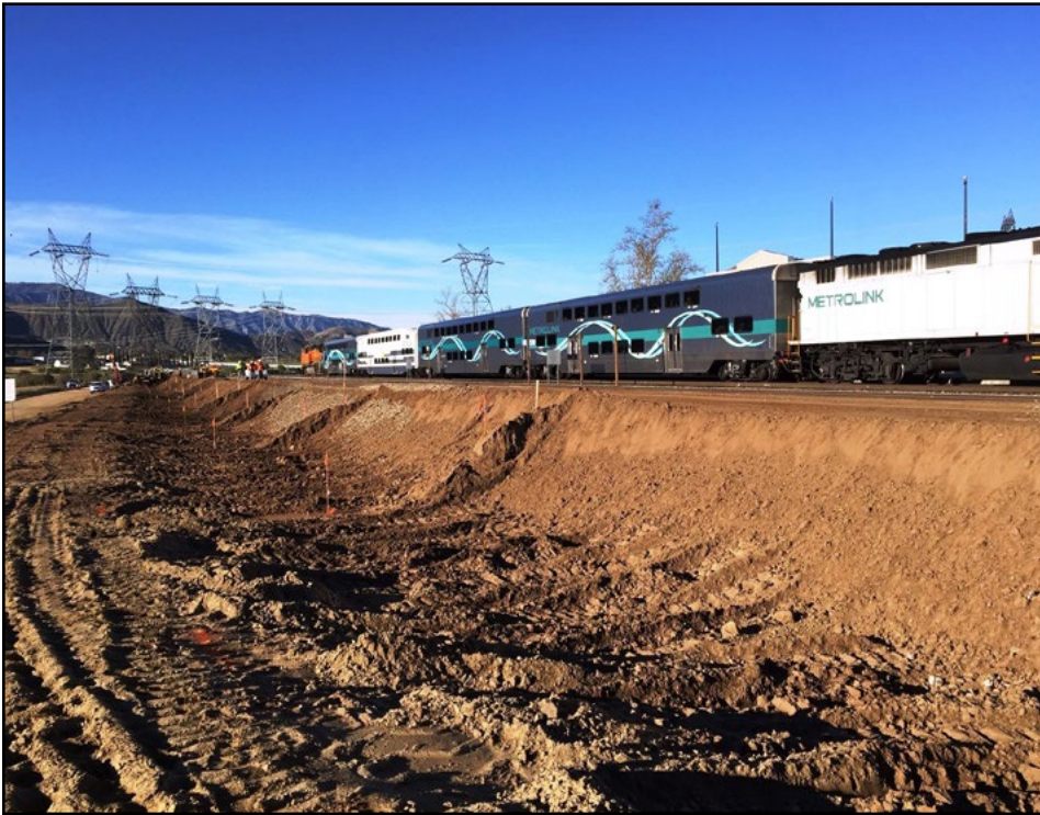
A built-up dirt pad for the new Vincent Grade Acton station platform sits directly across from the existing platform.
