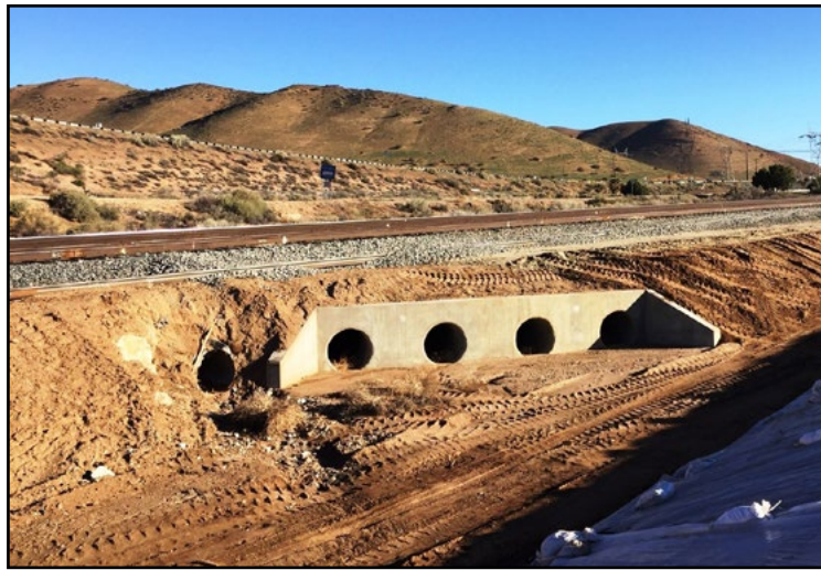
Rasmussen crews installed a four-barrel, 36-inch RCP culvert headwall running underneath newly laid tracks in order to carry storm-water runoff.
