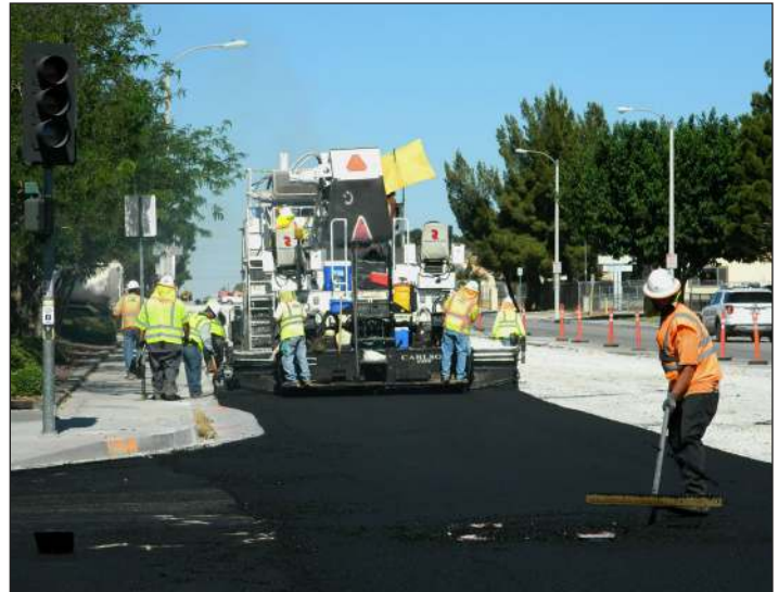
Rasmussen’s paving crew works along La Mesa Road in Victorville.
